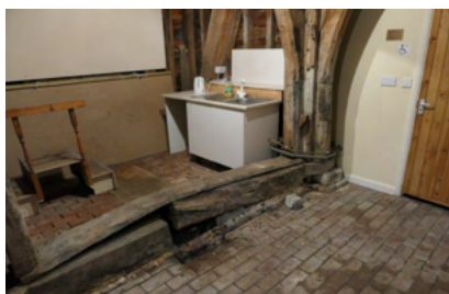
Rotted plate before work started
