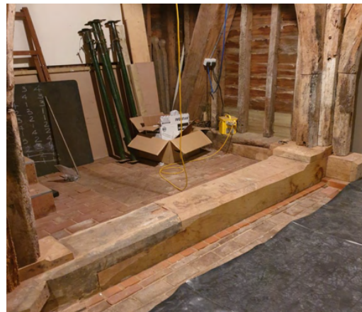
Rotted wood replaced south side
