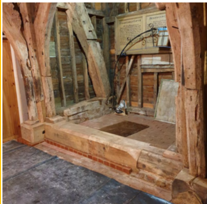
Rotted wood replaced on North side
